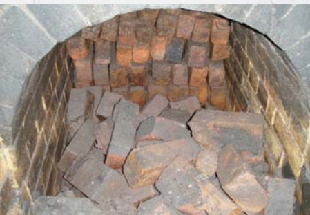
Stacked bricks in the flue beneath the aniline salts shed
