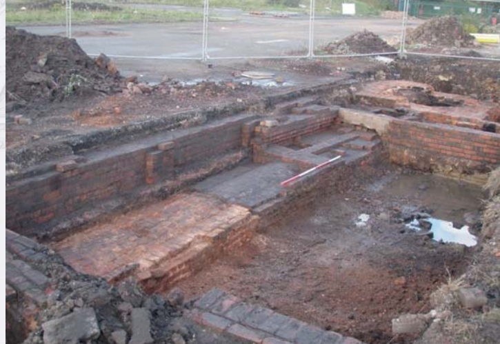
Excavated remains of the aniline salts shed, with the foundations for the chimney to the rear
