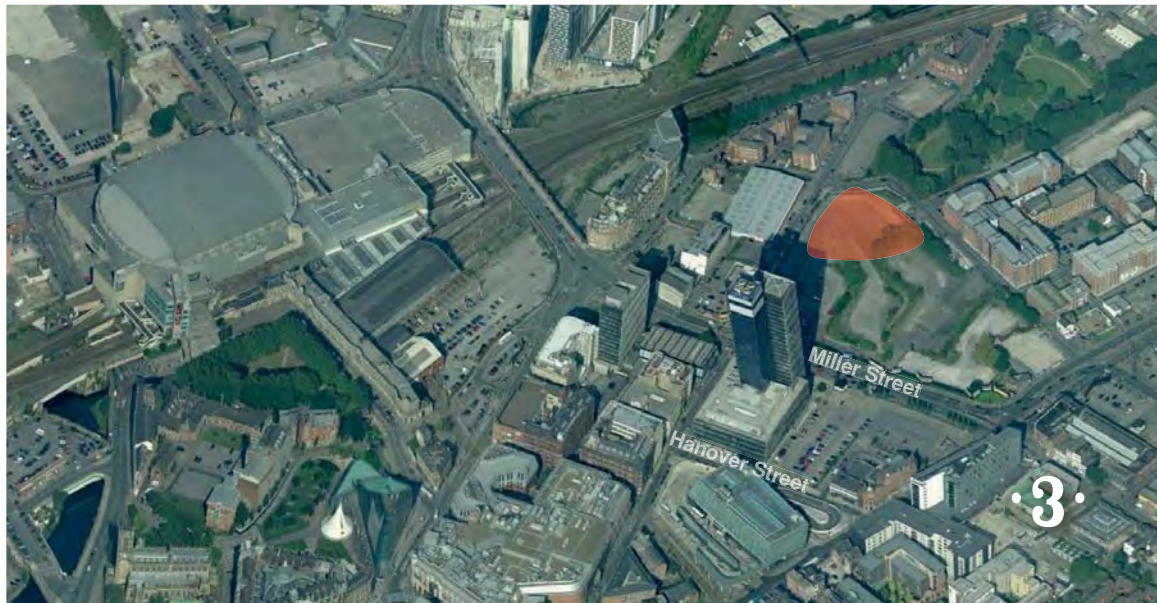
Aerial view across Shudehill in 2005, showing the footprint of One Angel Square. The construction of this iconic building in 2010-12 as part of the NOMA scheme has acted as a catalyst for the regeneration of the area
